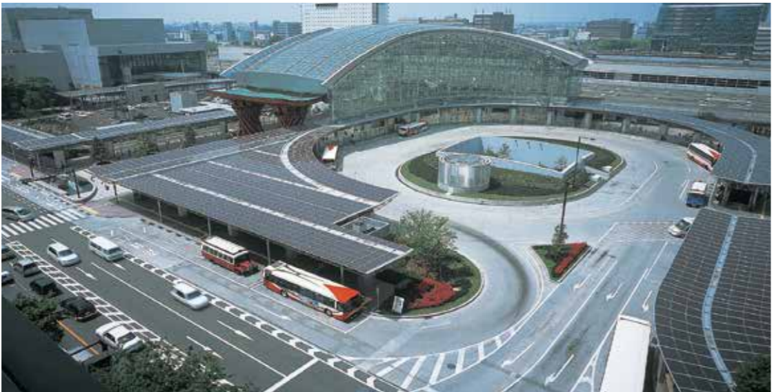
Kanazawa Bus Station BIPV Project
