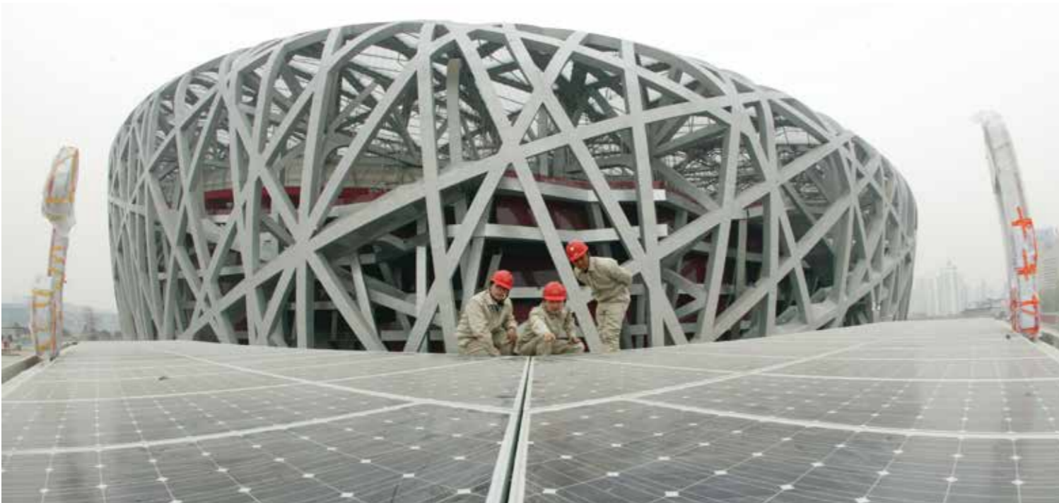
Beijing Bird's Nest Stadium BIPV Project
