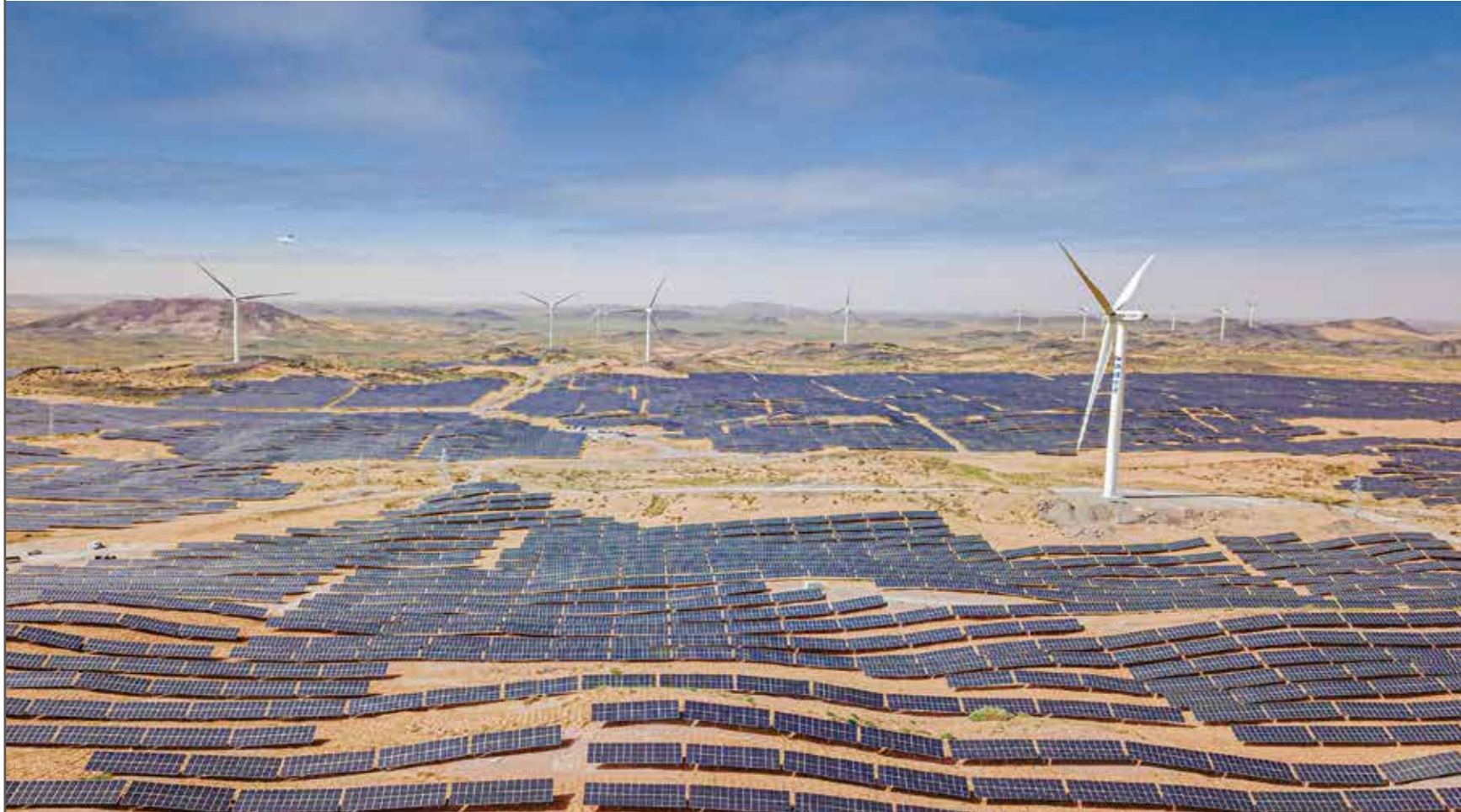
CDB New Energy Collected Ningxia Weigang, Yongning and Hongsibao Project in 2020
