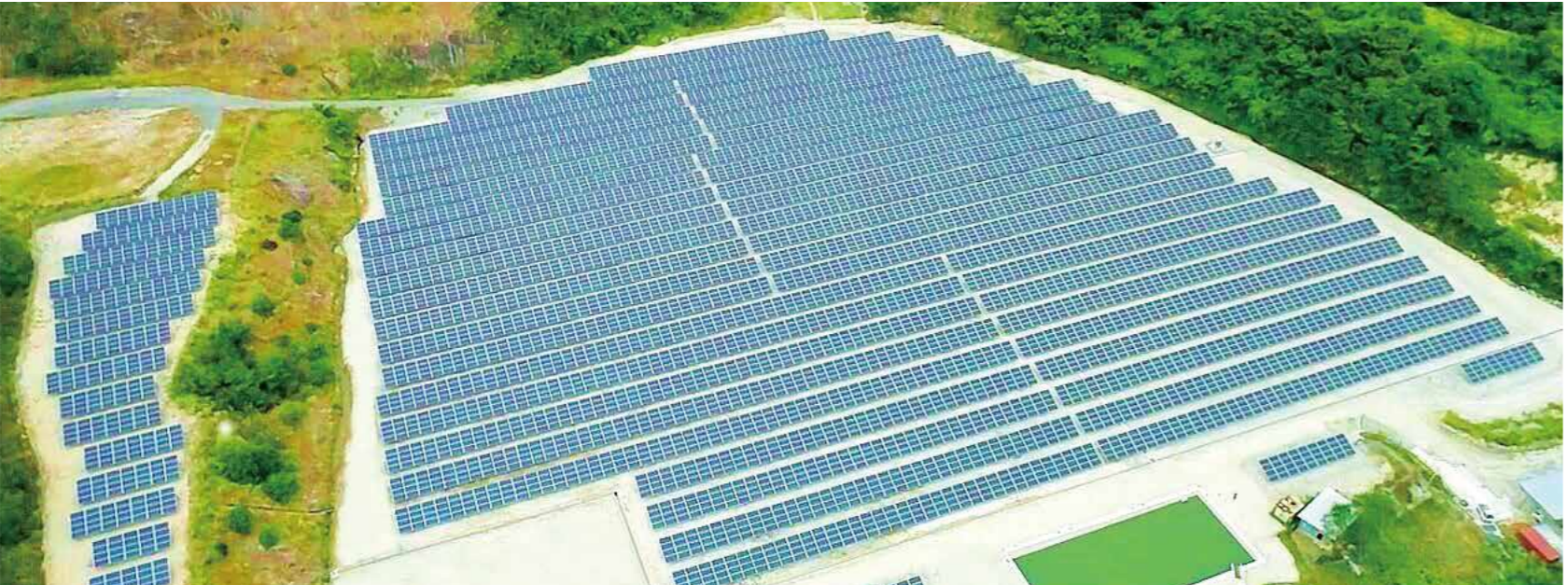
Japan 3.24 MW Power Plant Project Kanzaki Solar
